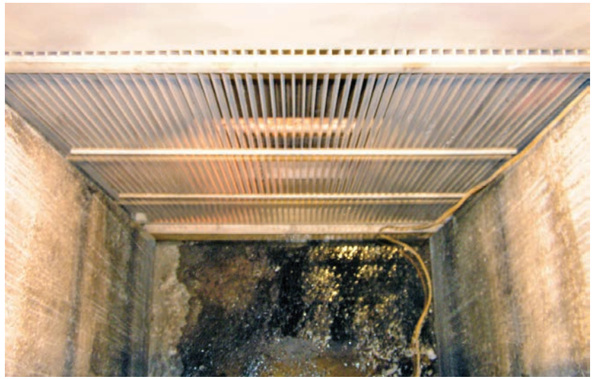
The screens have jam-resistant chain guides and bar racks with 1-inch openings.
