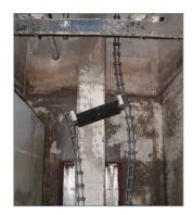
ABOVE: Broken plastic chain on grit collector
