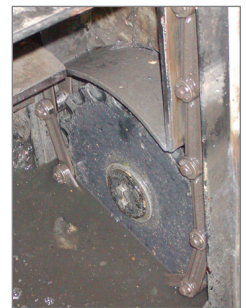
DuraMax cast stainless steel chain and urethane sprockets newly installed in 2005 (above); and same today (below) looking hardly any different.
